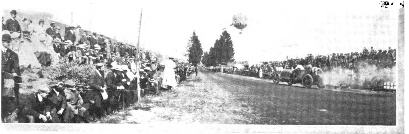
GENERAL VIEW IN THE VICINITY OF THE GRANDSTAND—NOTE EXCELLENT ROAD WHICH STRETCHES AWAY INTO THE DISTANCE.
